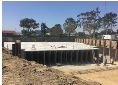
Pre-Cast Subsurface Infiltration Facility
