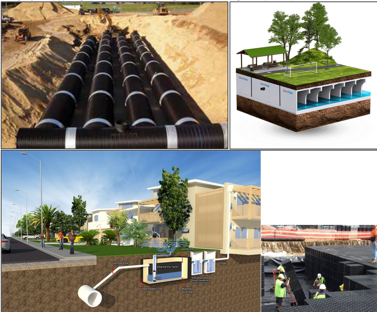
Figure 1 – Contech DuroMaxx Underground Water Storage Tank (upper left); StormTrap™ SingleTrap® Concrete Underground Storage System (upper right); Atlantis Flo Tank Underground Water Storage Tank (bottom).
